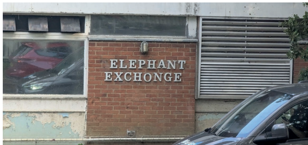
Signage wordplay on a sorry-looking redundant telephone exchange in Ottershaw, Surrey
